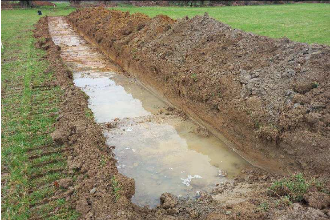
Plate 15: View of the area of the large land drain revealed at the west-south-western end of T.6
