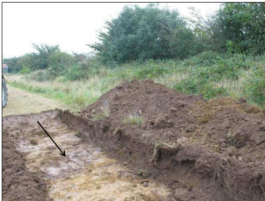
Plate 6: View of section along edge of south field boundary with land drain indicated
