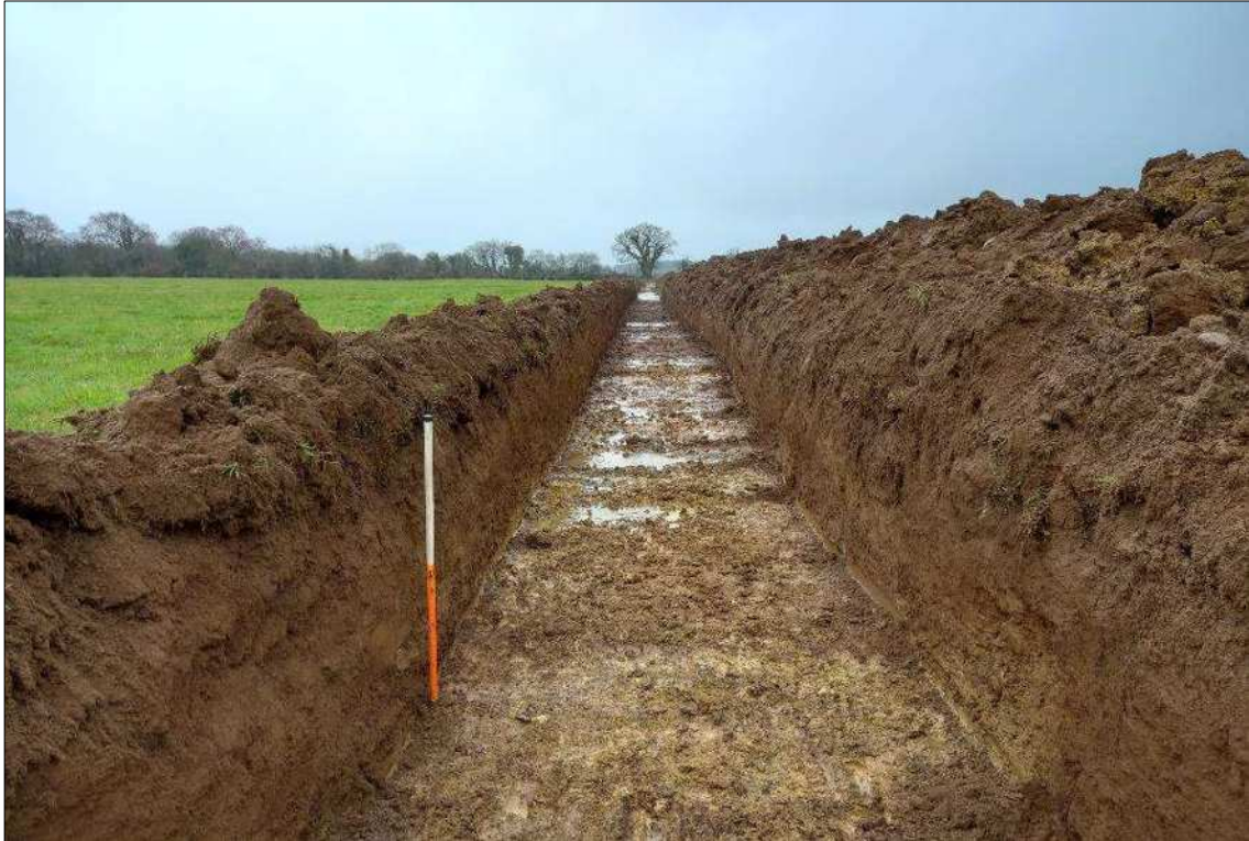
Plate 17: View to west-southwest along the excavated T.6
