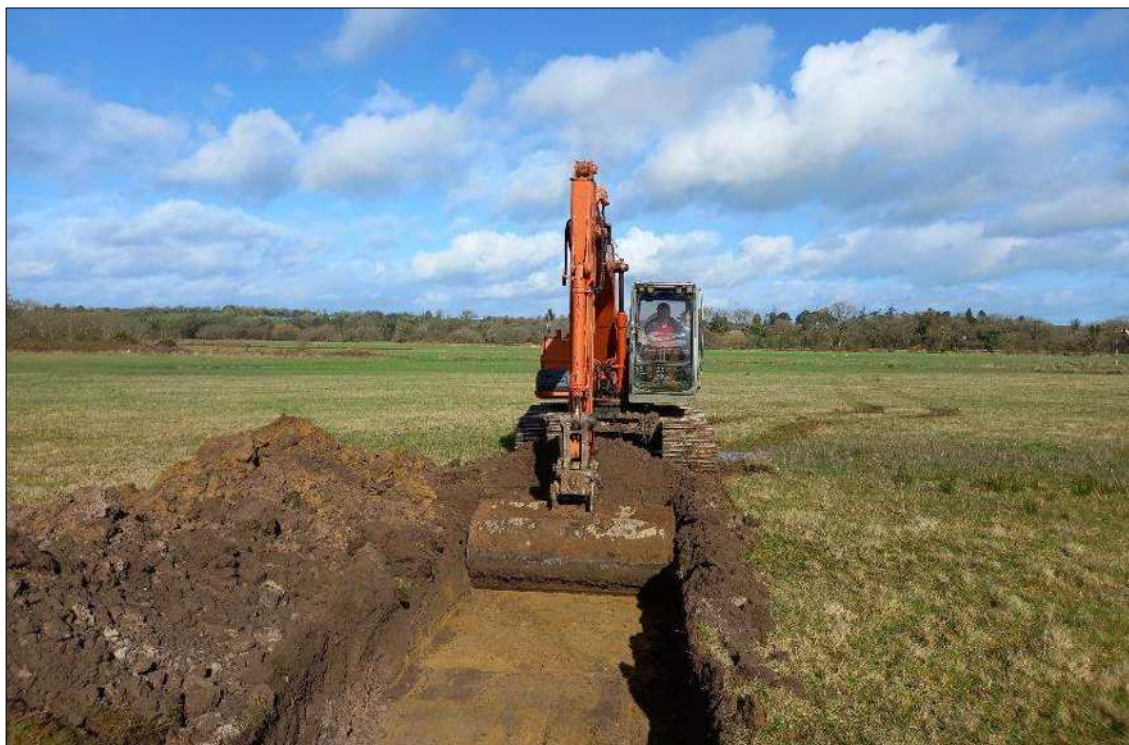
Plate 1: Trenching commences in Trench 1, facing northwest
