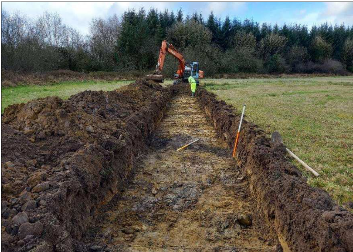
Plate 4: View of the excavation of T.2 in progress, land drain evident in centre of frame, facing southwest
