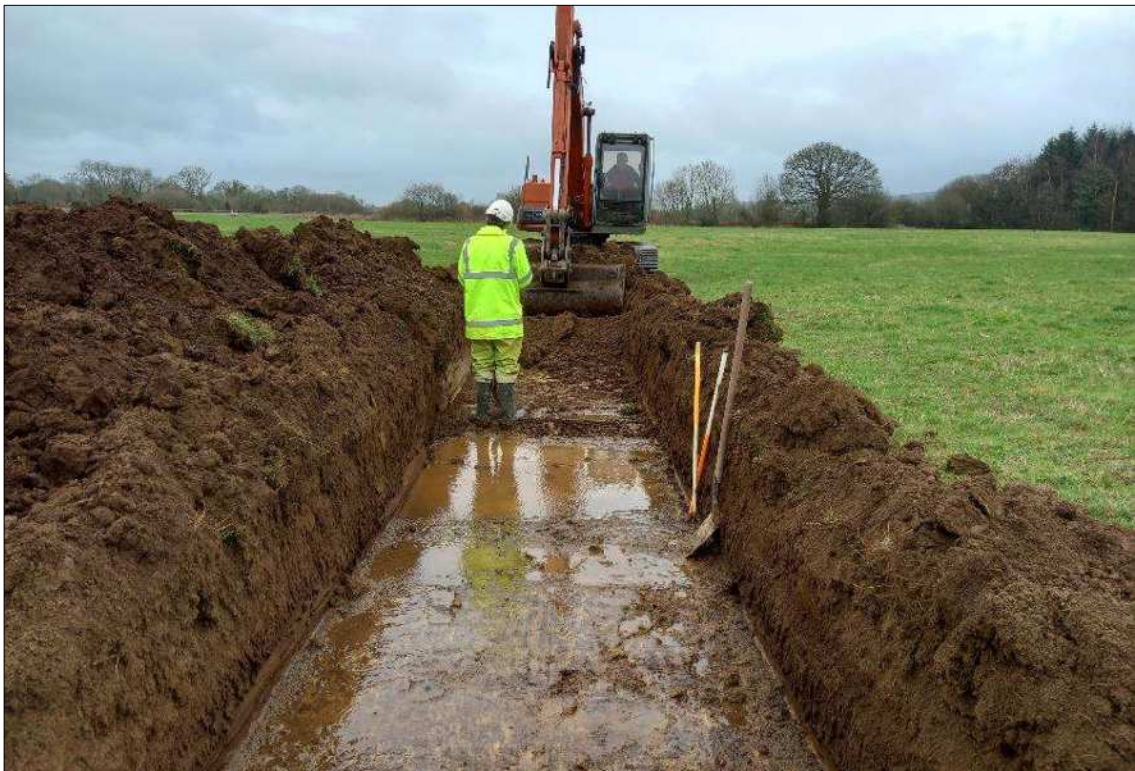
Plate 14: View of the excavation of T.6 in progress, facing west-southwest
