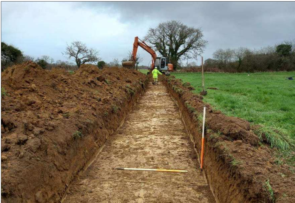
Plate 18: View of the excavation of T.7 in progress, facing east-northeast
