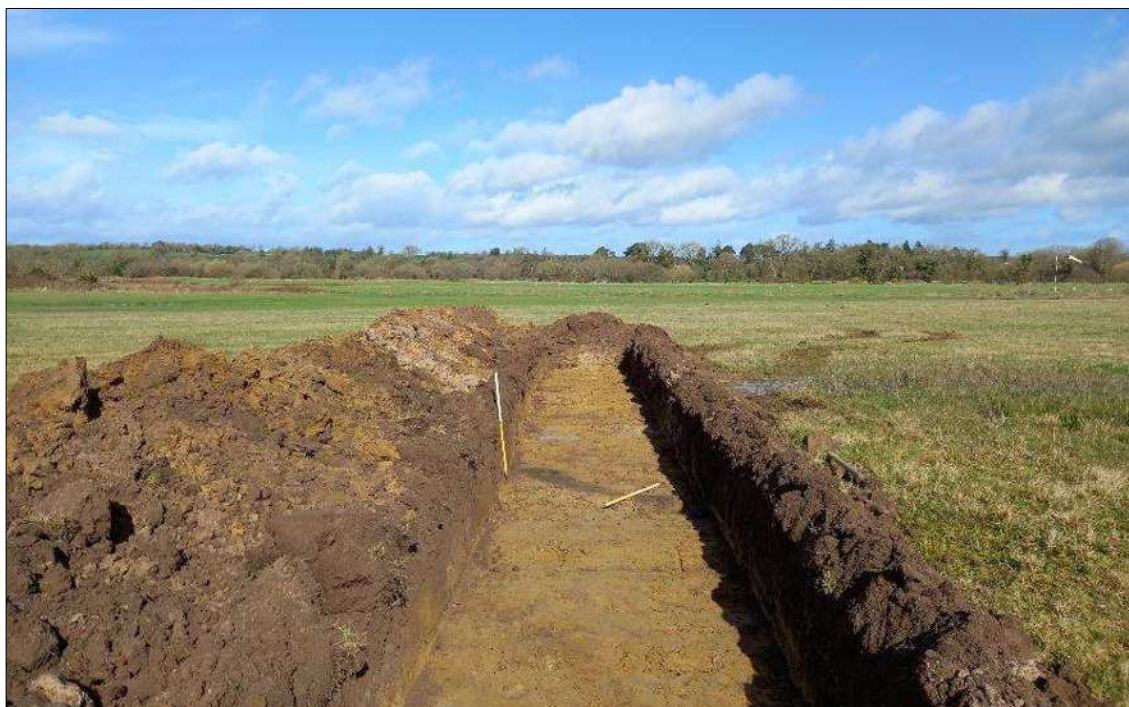
Plate 2: View across T.1, land drain evident in centre of frame, facing northwest
