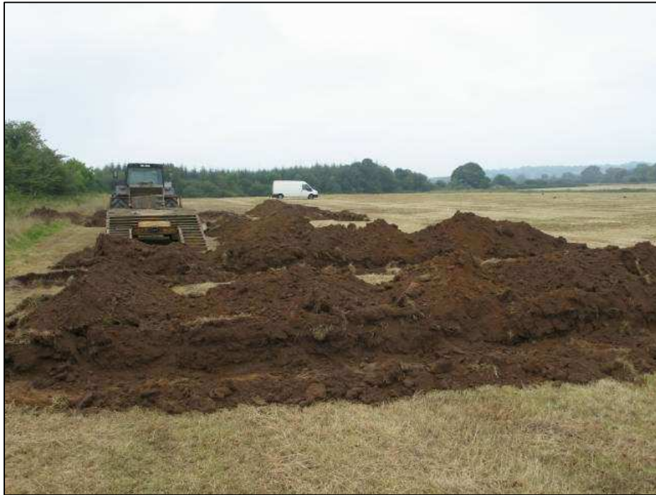
Plate 3: General view of test trenching from east
