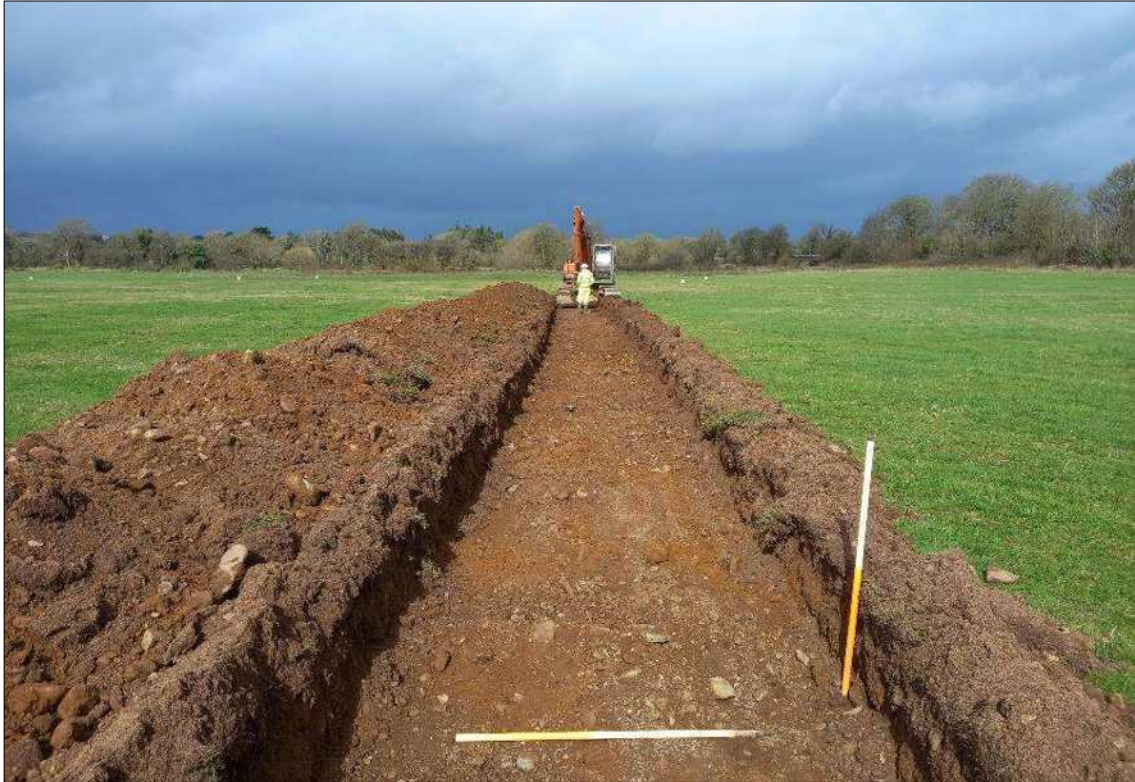
Plate 9: View of the excavation of T.4 in progress, facing north-northwest
