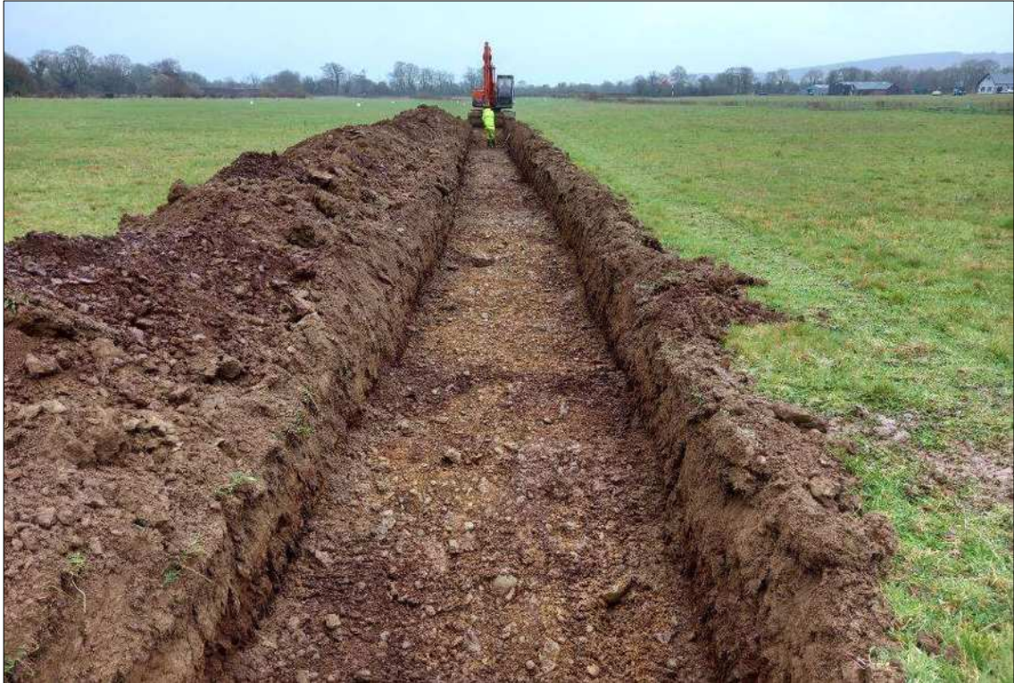
Plate 11: View of the excavation of T.5 in progress, facing east-northeast
